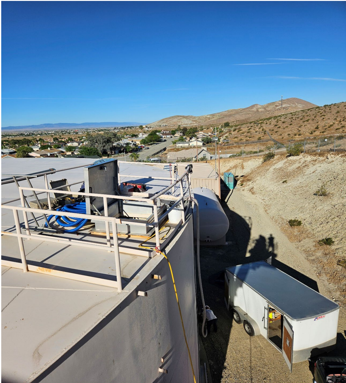
Tank inspections in progress , divers at work.
