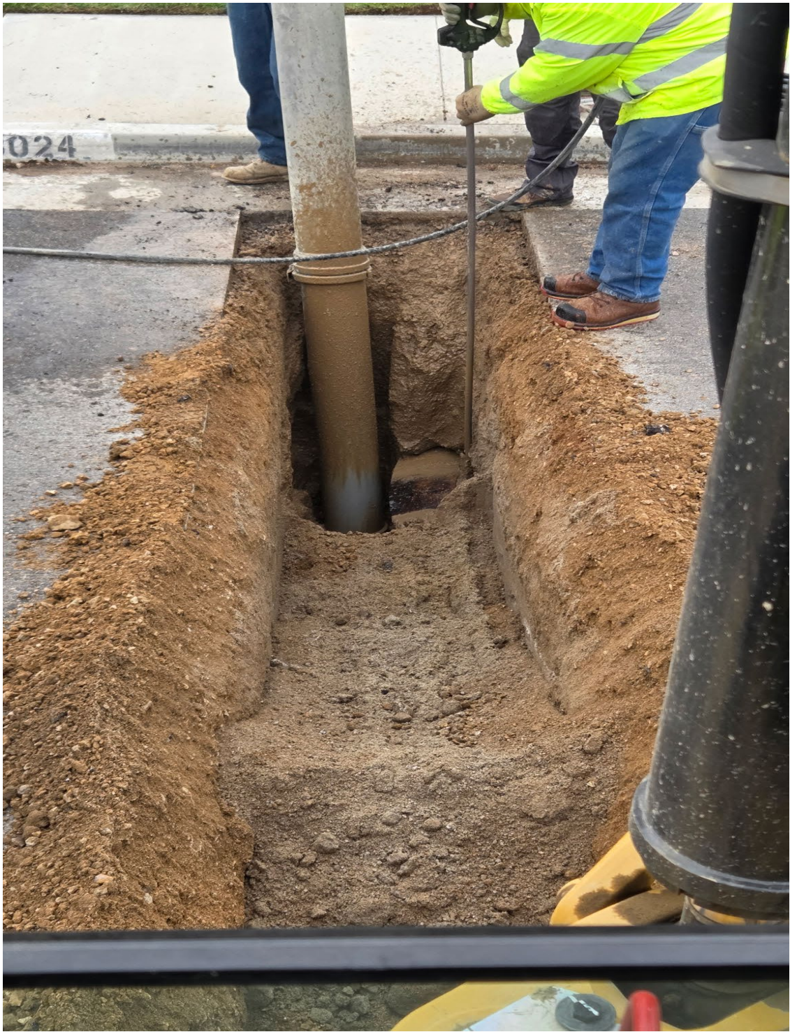
Locating corp stop to shutoff in preparation for service line replacement.
