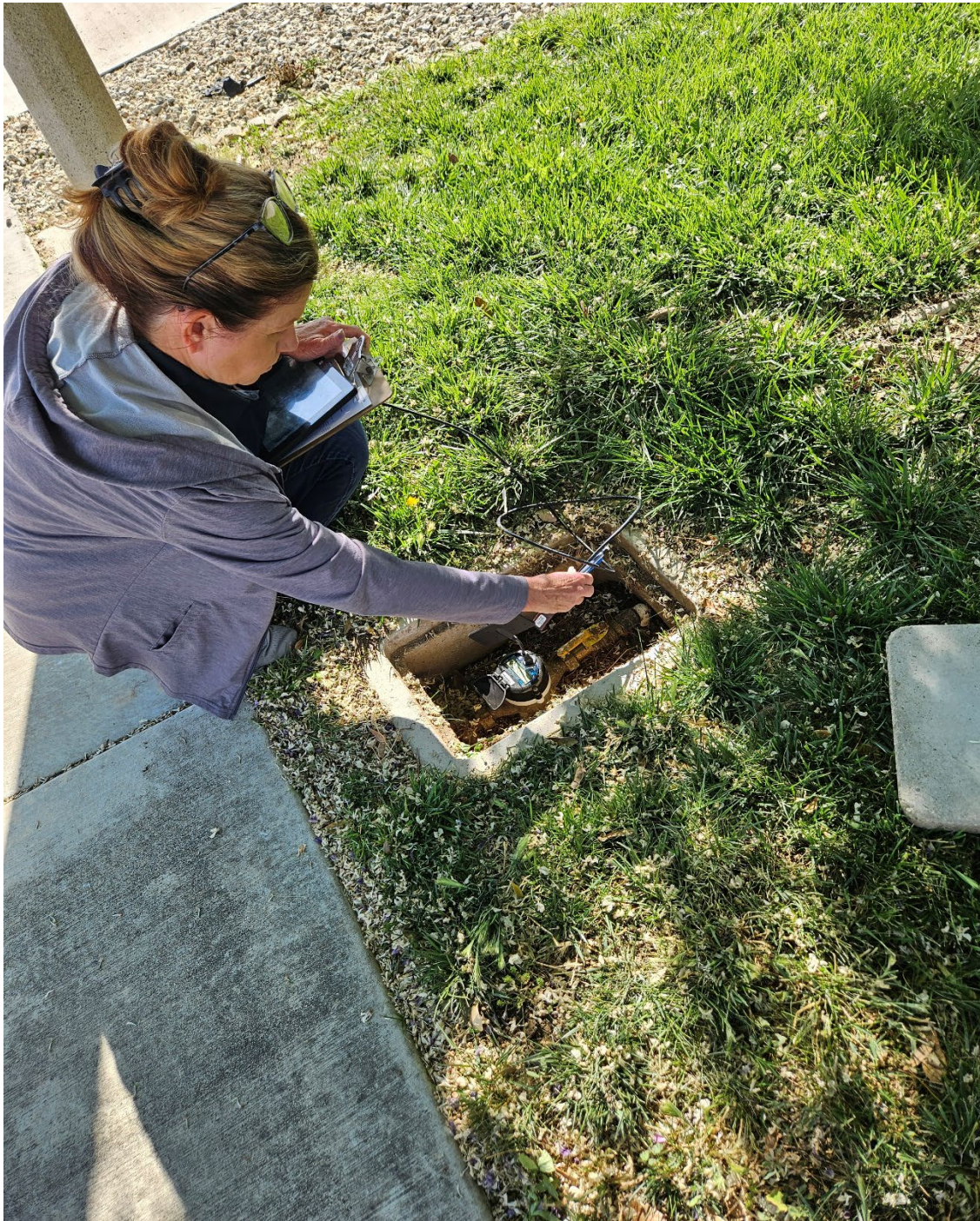
Public works staff sending a chirp to an uncommunicating Metron register
