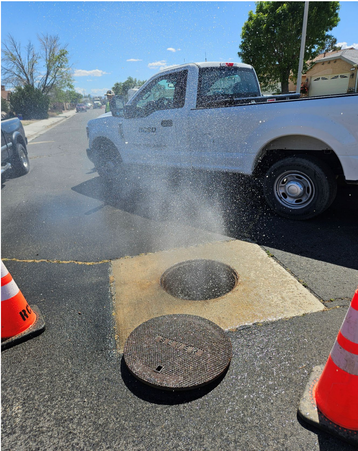
Sewer jetting in progress , warthog jetter nozzle reached desired manhole
