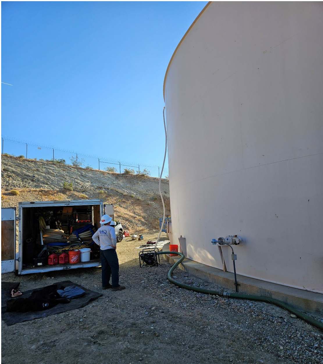
Tank divers getting ready to dive in tank 4 for inspections
