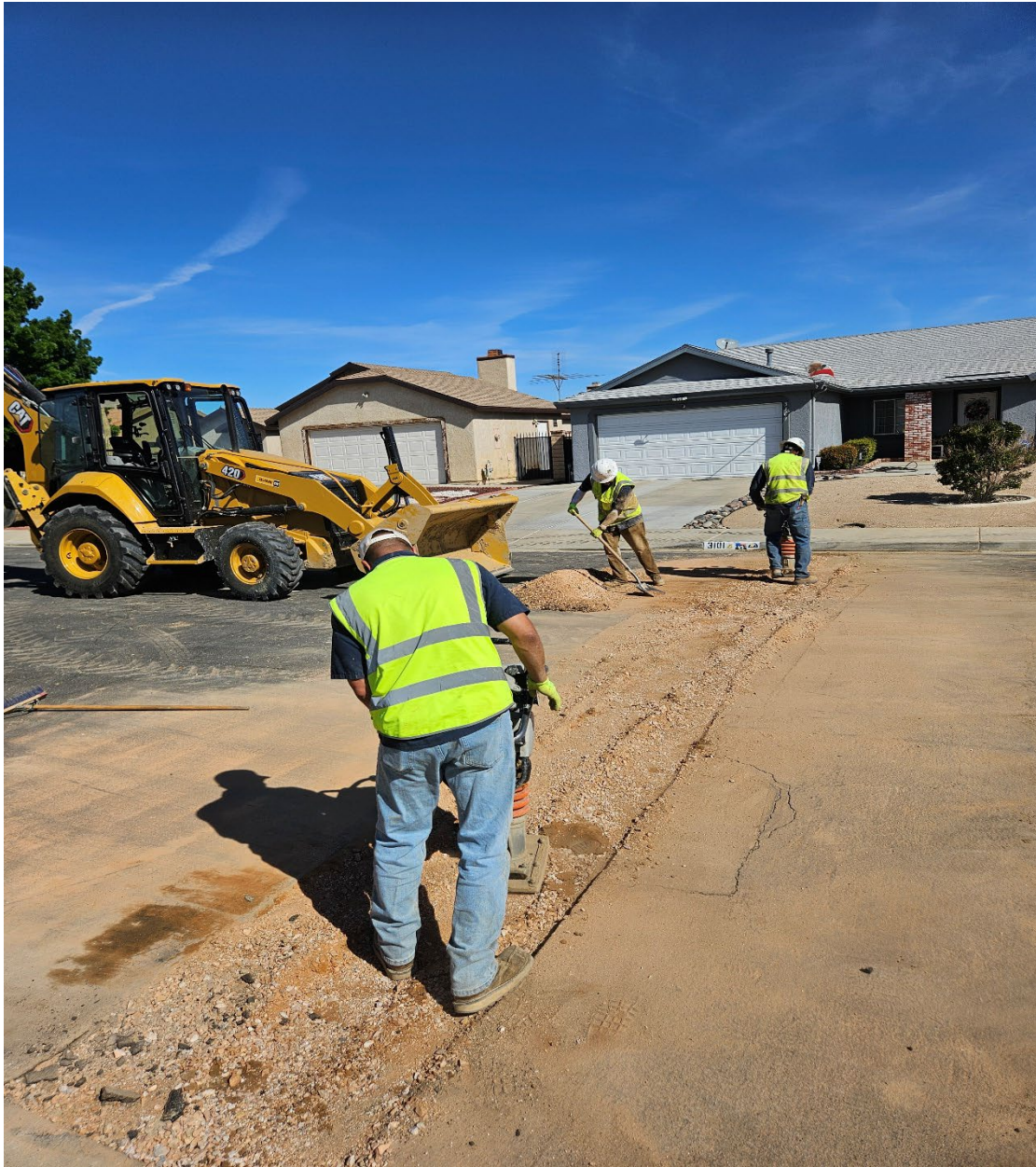
Richland service line replacement complete, backfill and compaction.
